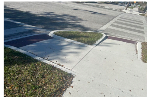
ADA Curb Ramp with Detectable Warning
