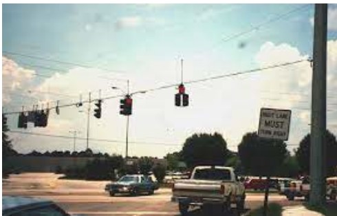
Replace Span Wire with Mast Arms
